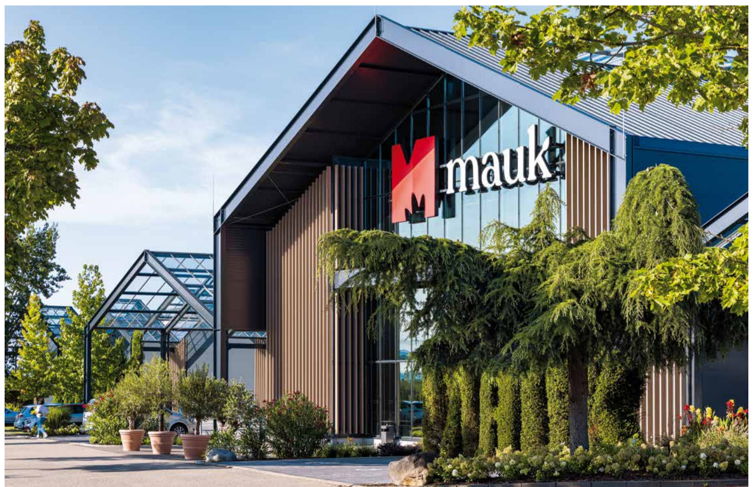
Mauk experience garden center successfully upgraded during ongoing operations.
